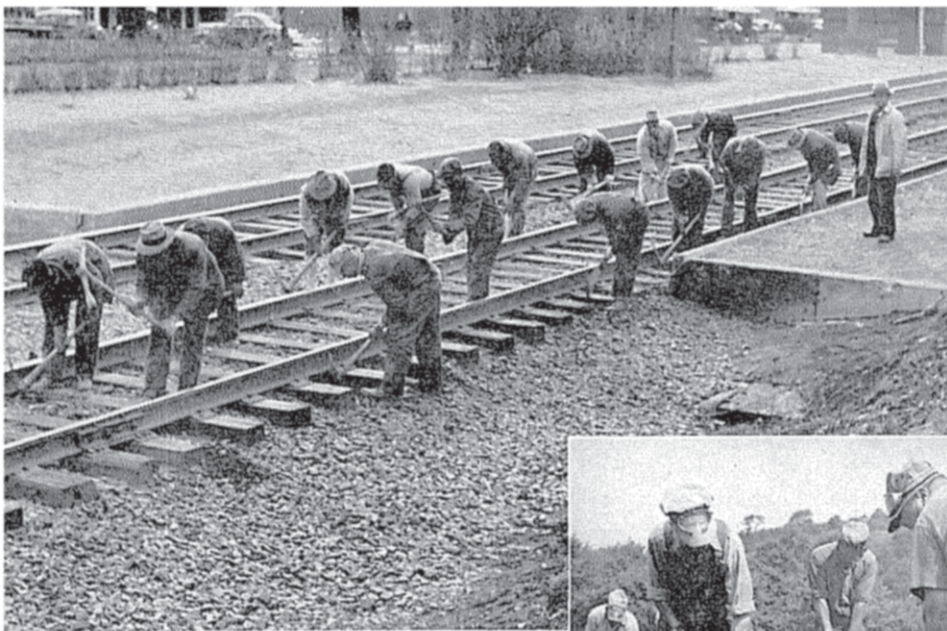
↑ Above: A gang of men surface track with hand tools under the direction of their foreman.
