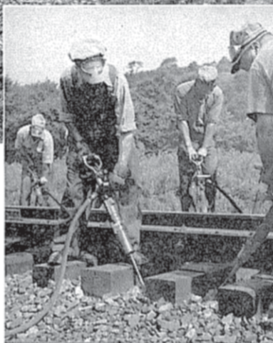
↑ Above: A gang of men surface track with hand tools under the direction of their foreman.
