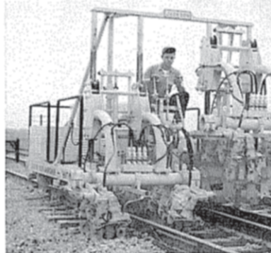
Right: This modern mechanical tamper requires the services of a skilled operator.
