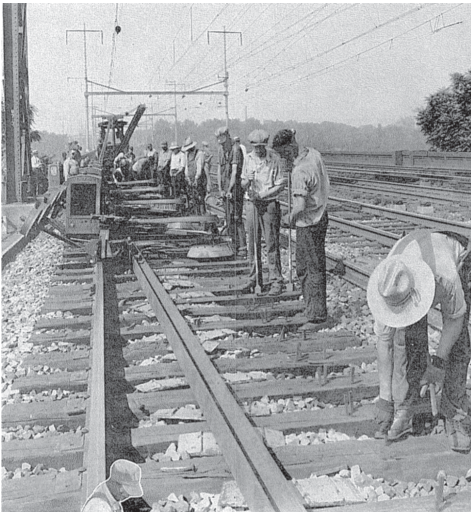
↑ Above: A rail-laying gang at work. After the spike holes have been filled with wooden plugs, ties will be resurfaced by the adzer in the background.
