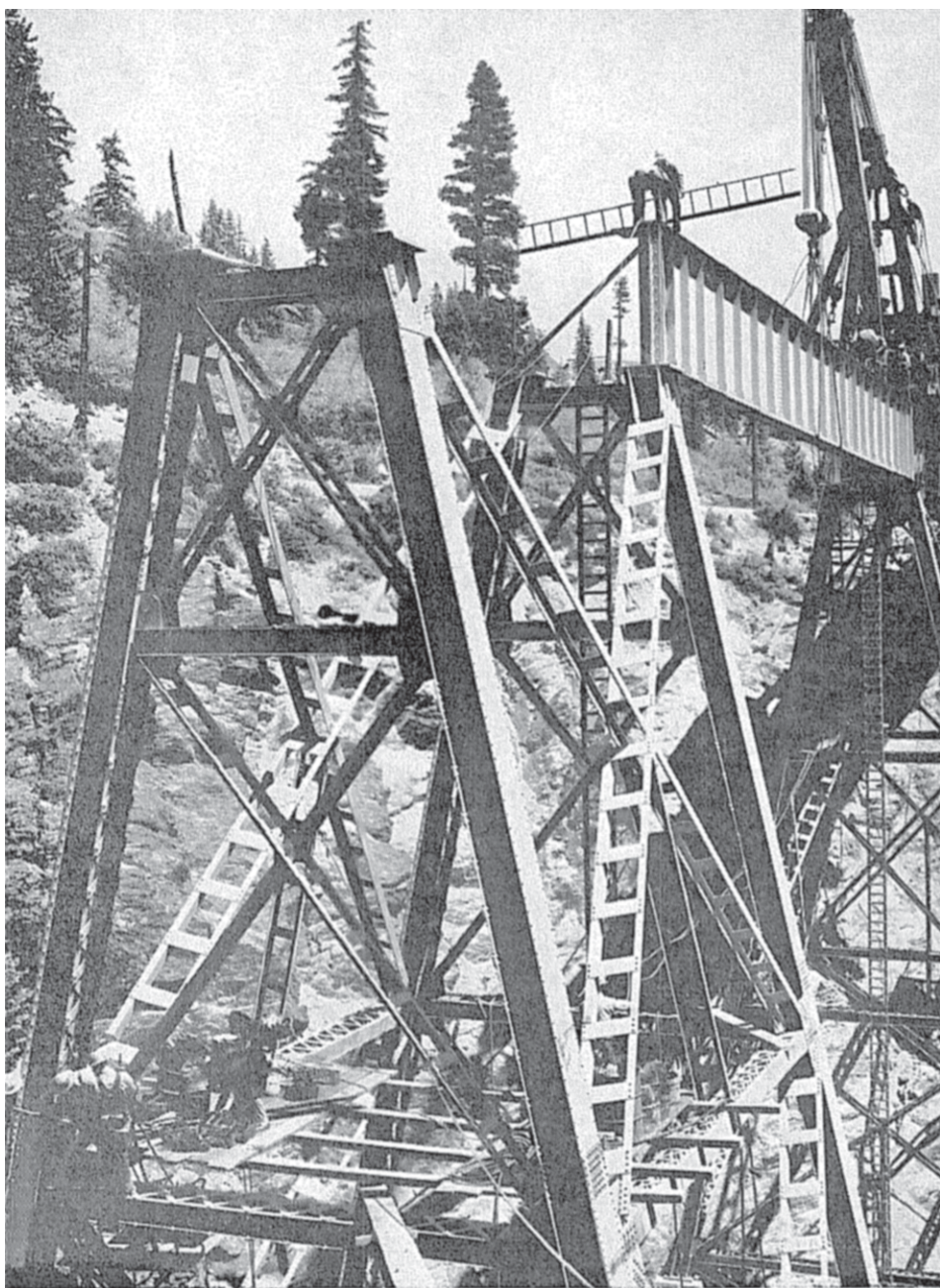
Above: A bridge under construction on the Great Northern Railway to be maintained by maintenance of way workers. The job of lowering the 37-ton girder took three and one-half hours.
