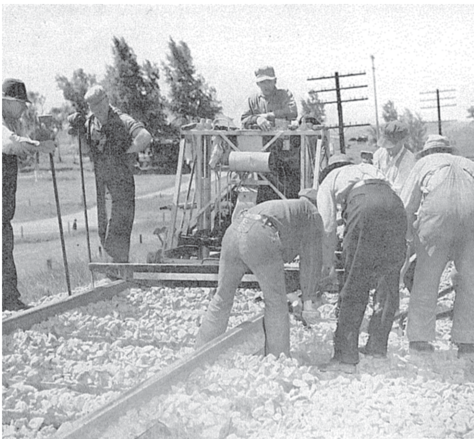
↑ Above: The power track jack is being used to raise track in a surfacing operation.
