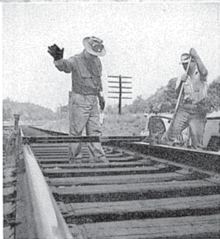
Right: The picture illustrates the use of hand jacks under the alert eye of the foreman.
